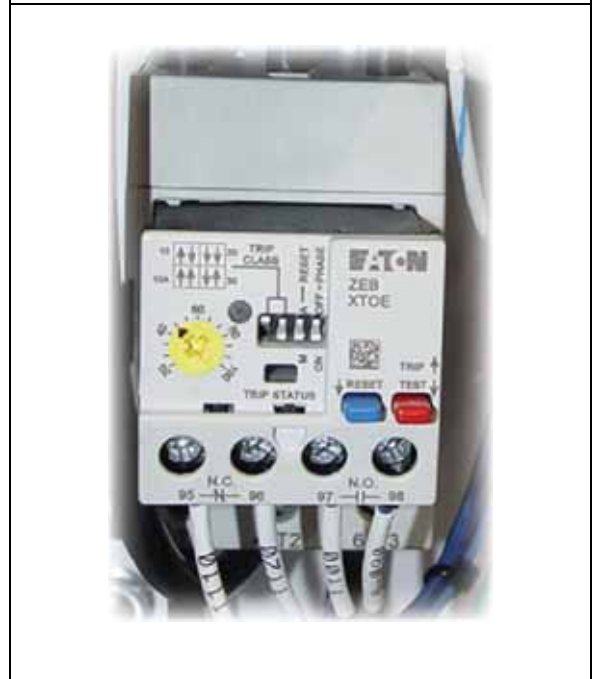
Figure 6-7 Overload Relay (typical)
